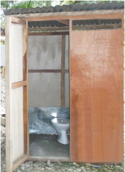
Members can choose between bamboo, plywood, or concrete outhouses, depending on their budget. All toilets come with a porcelain flush bowl and a septic tank.
